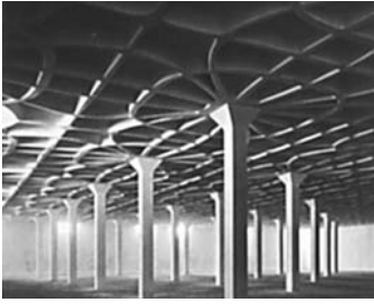
Fig. 5: The Gatti wool factory ceiling structure
